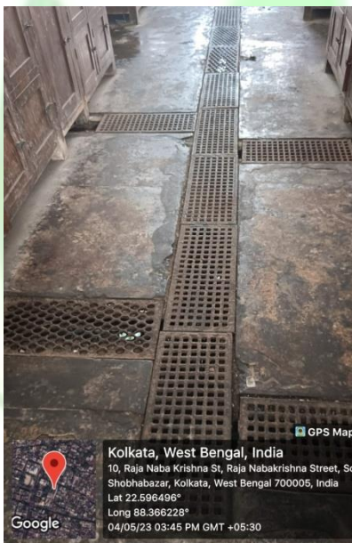
Drainage in Laboratory
